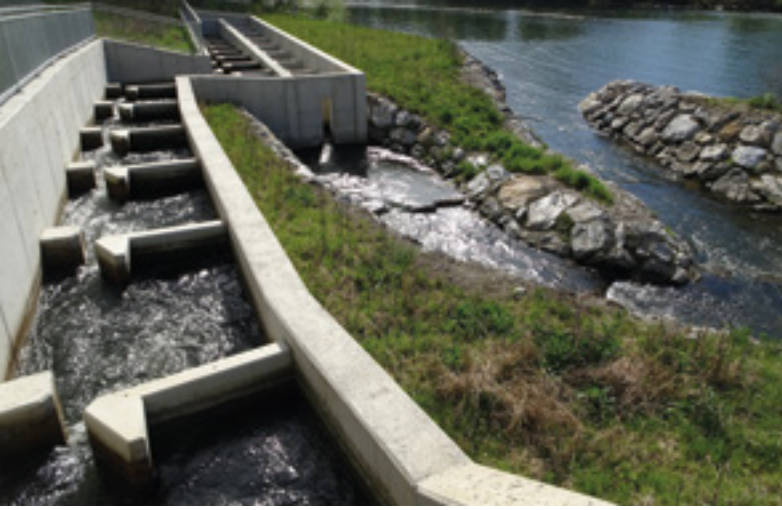
Abb. 7: Schlitzpass - KW Peggau - Mur © Schmid / IB Parthl
